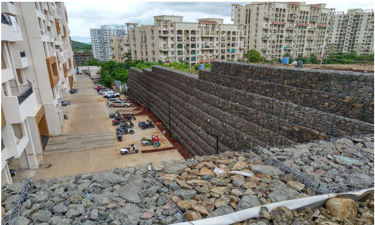
RE wall With Gabion facia.
