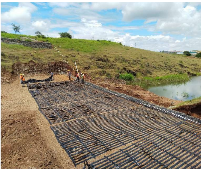
Paralink (100 Grade) Laying
