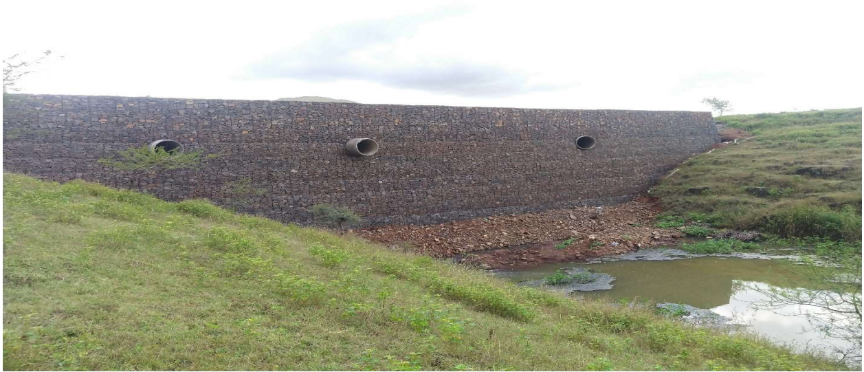
12 m. Height RE wall With Gabion facia.
