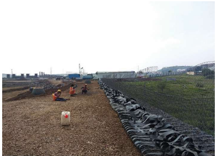
4mX2mX1m Terramesh Unit Installation
