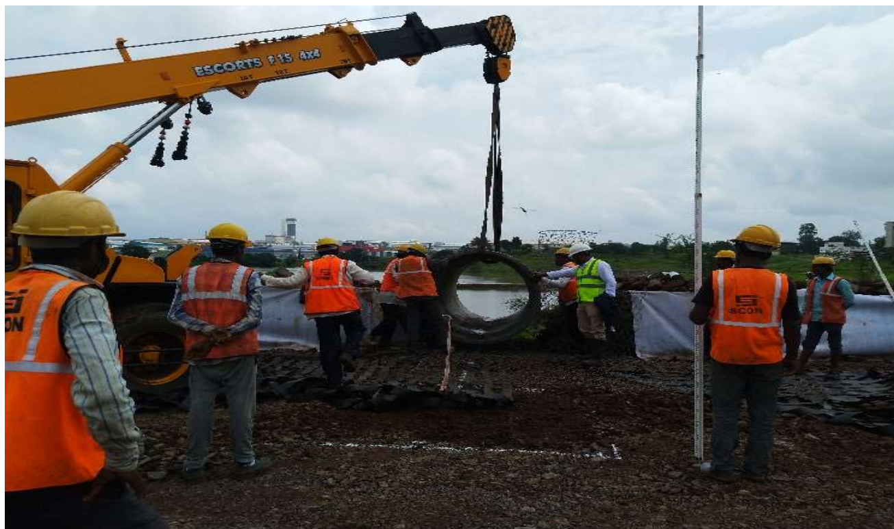
LAYING OF SWD PIPE 1200MM DIA
