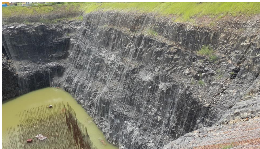
Completed works for Slope protection works
