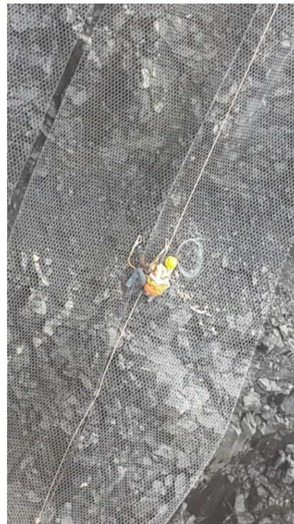
Climber carrying out the lacing of adjacent netting panels
